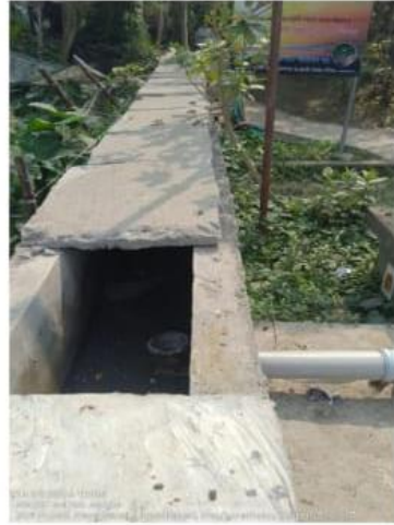
Grey water comes into settler tank
