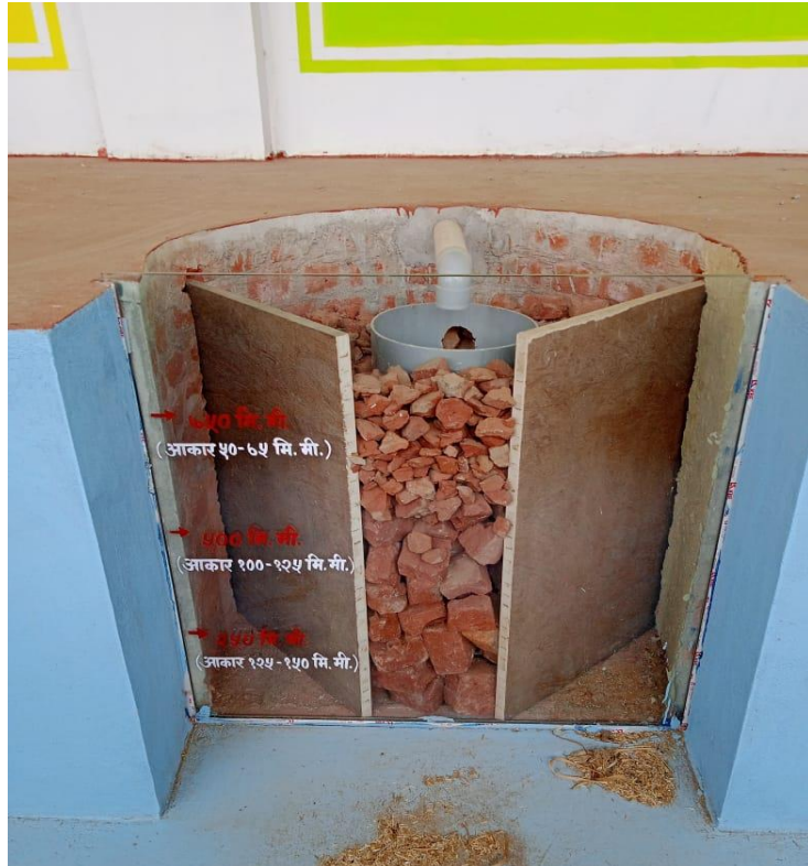
Magic Pit 1 m (depth) x 1 m (diameter)
