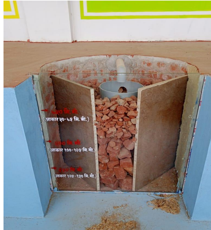
Modified Magic Pit 1 m (depth) x 1 m (diameter)
