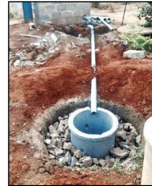
Construction of Magic pits in Telangana
