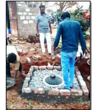
Construction of Magic pits in Telangana
