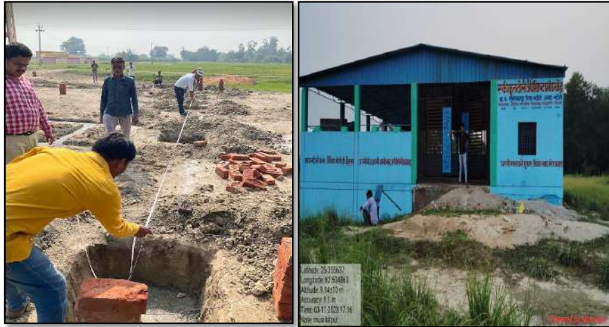
Construction of Resource Recovery Centres in UP
