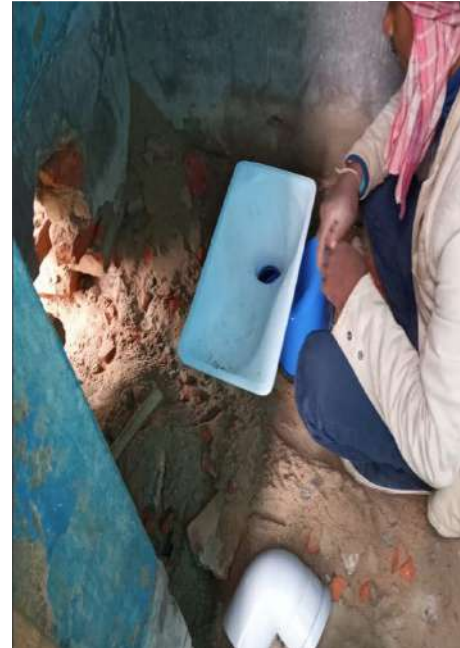
Retrofitting in progress
