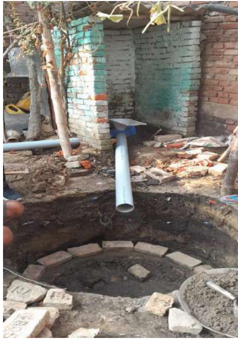
Converting single pit to two pit
