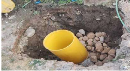
Soak pit & Magic pit Demonstration at Jammu
