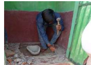
Retrofitting in progress
