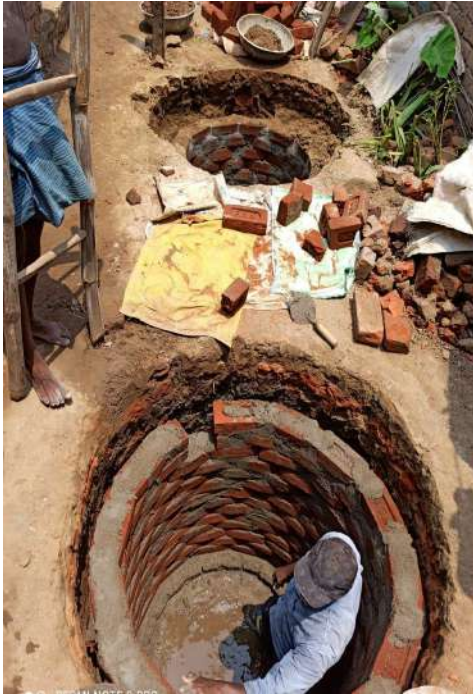
Retrofitting in progress
