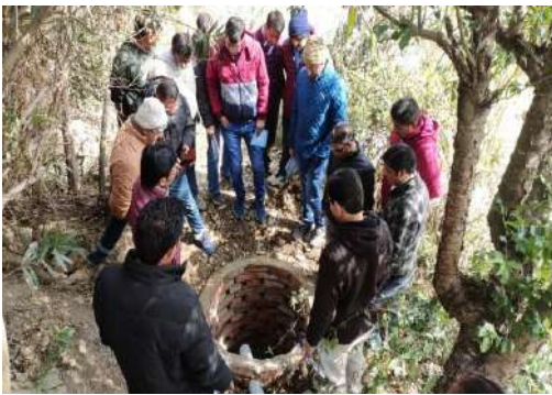
Toilet retrofitting demonstration at HP
