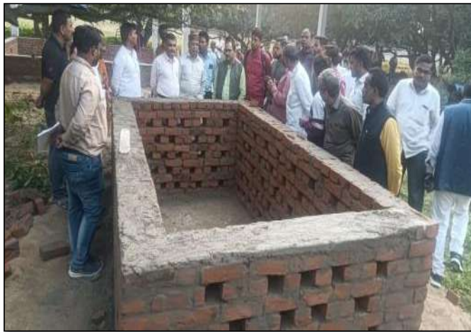
Demonstration of NADEP construction in UP
