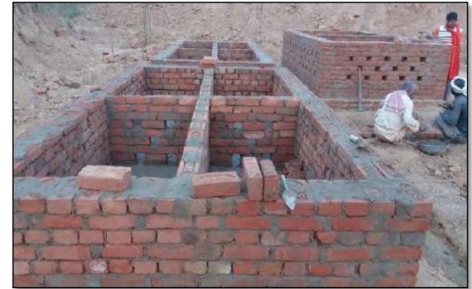
Construction of vermicomposting pit in UP
