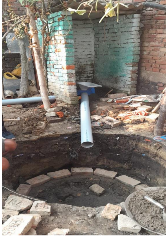
Converting single pit to two pits
