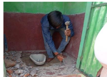
Retrofitting in progress
