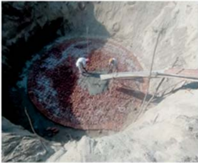
Laying of foundation
