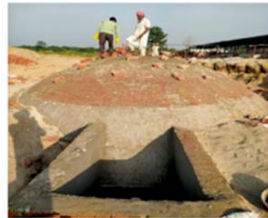
Construction of dome & bigger portion of outlet chamber
