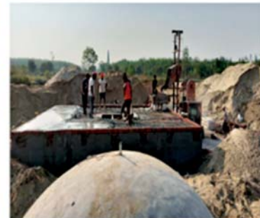
Completion of bigger portion of outlet chamber
