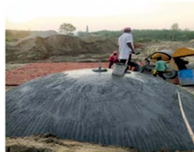
Completion of dome
