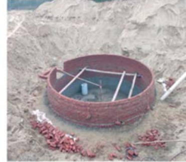
Construction of dome
