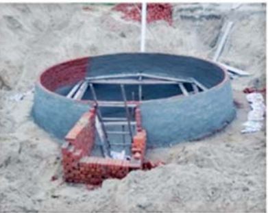
Construction of smaller portion of outlet chamber
