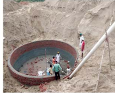
Installation of inlet pipe
