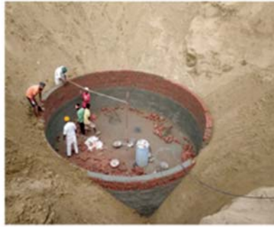
Construction of digester
