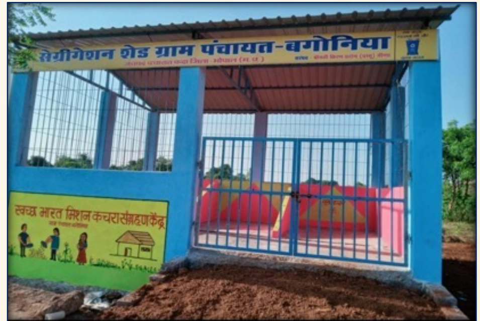
Segregation Shed constructed at GP Bagonia of Phanda Block
