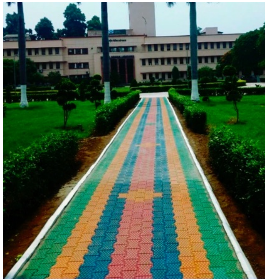
Floor tiles made from a mix of HDPE, PP and LDPE . The tiles are anti-static, antimicrobial, & anti-bacterial. They can also sustain heat up to 140°C & cold up to -25°C. A kg of plastic waste makes 1 sq ft of tiles which comprises of 4 plastic paver tiles.
