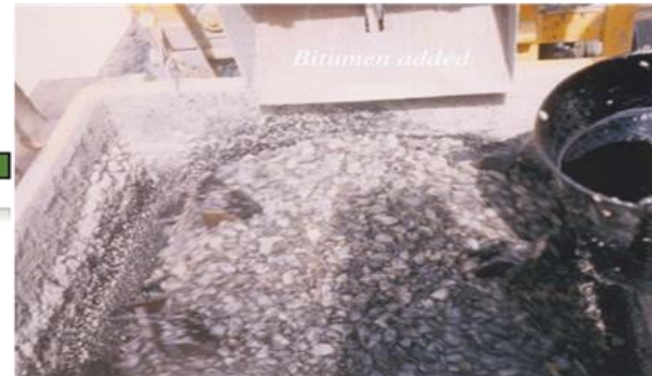
6. Addition of Bitumen
