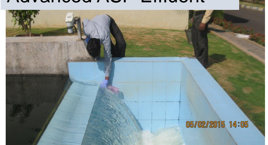
Advanced ASP Effluent
