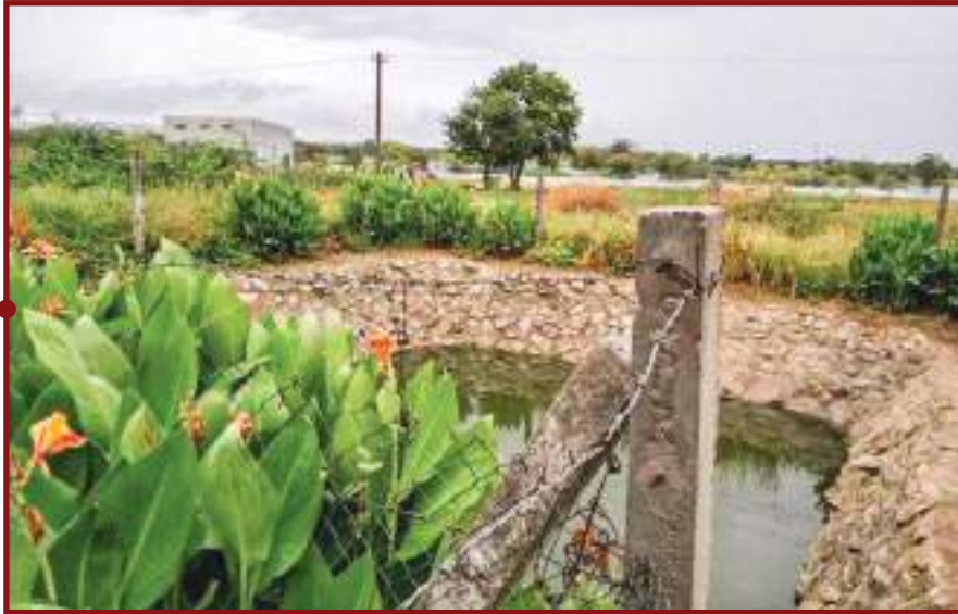
Image L: Polishing Pond of DEWAT System
