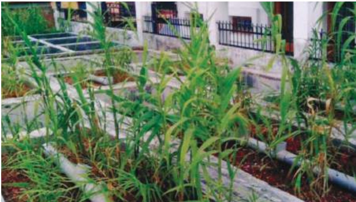
Image 4: Constructed Wetland at Village Level
