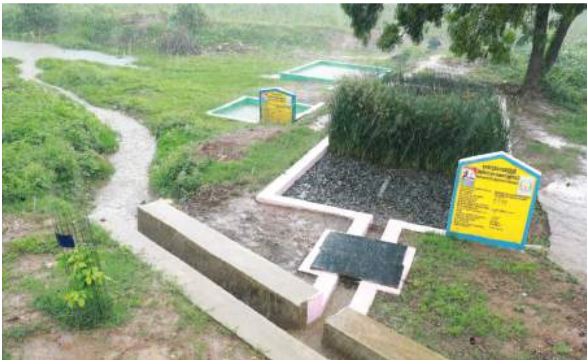
Image 9: Community Horizontal Filter System
