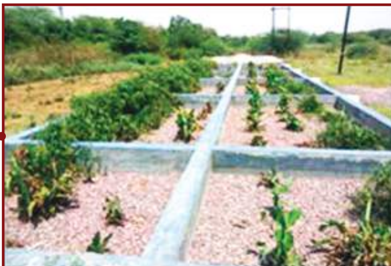
Image K: Phytorid Plant Constructed at Dhorka, Haryana
