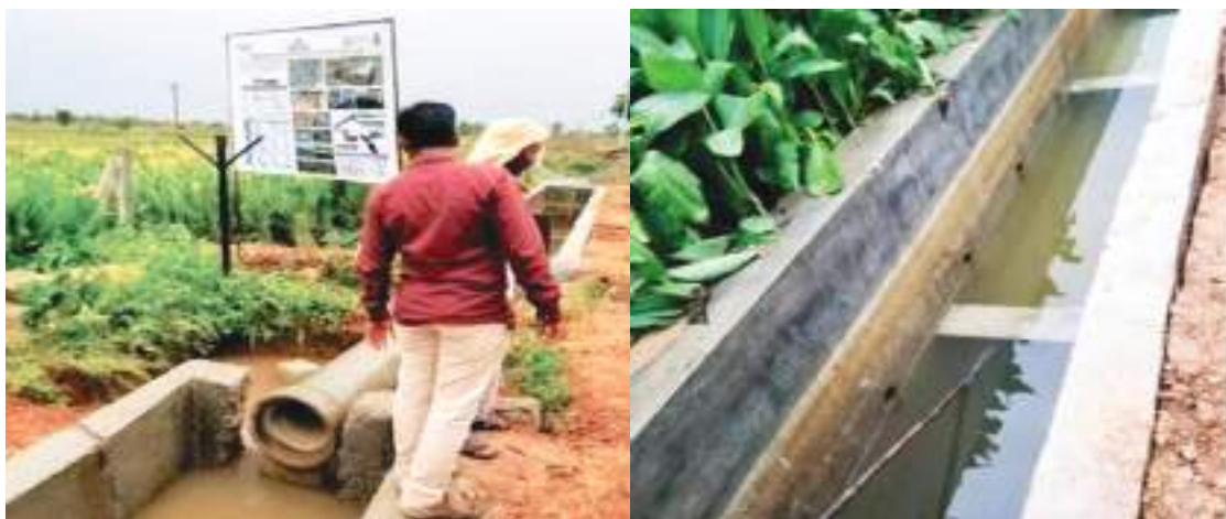
Image M: Equalization Chamber and Aerobic Baffled Reactor
