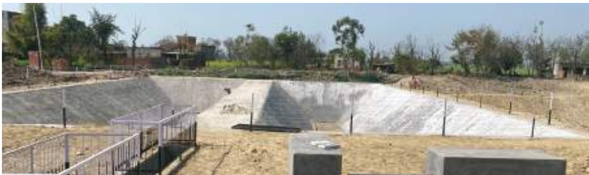
Image 3: WSP being Constructed
