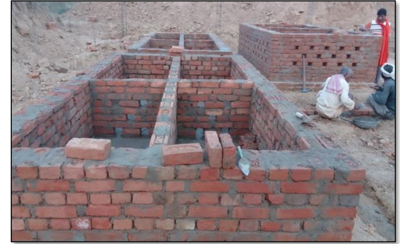
Construction of vermicomposting pit in UP
