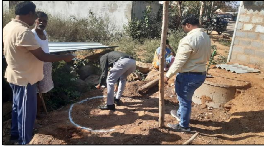
Site selection for Retrofitting of toilet single pit to twin pit in Telangana
