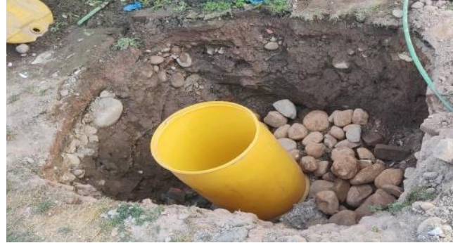
Soak pit & Magic pit Demonstration at Jammu
