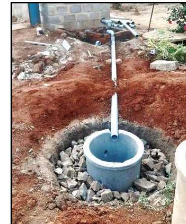
Construction of Magic pits in Telangana
