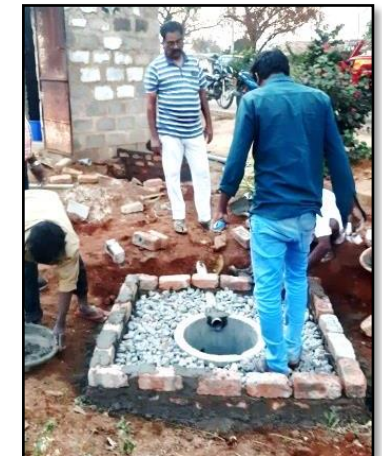
Construction of Magic pits in Telangana
