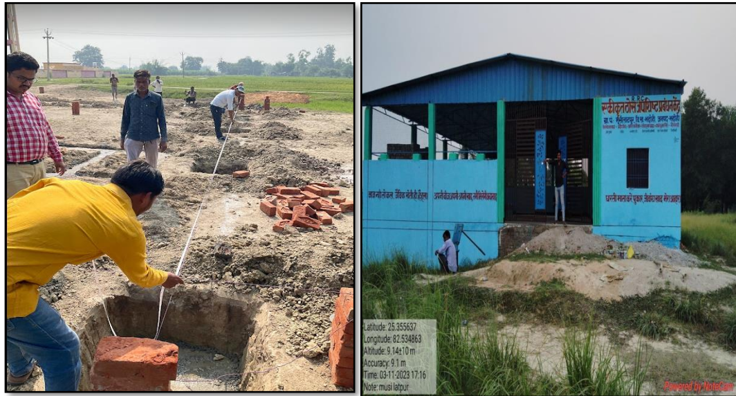
Construction of Resource Recovery Centres in UP
