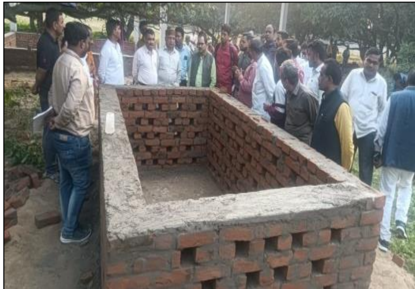
Demonstration of NADEP construction in UP
