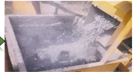
4. Aggregate transfer to puddler
