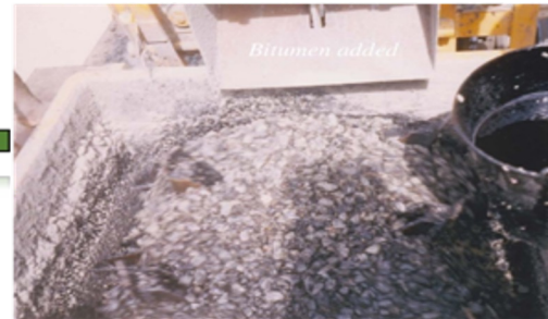
6. Addition of Bitumen
