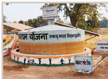
Bio Gas plant
