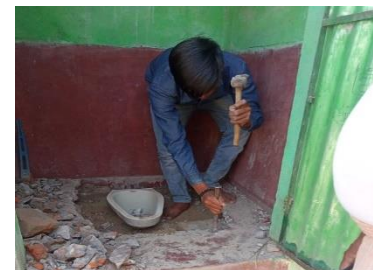
Retrofitting in progress
