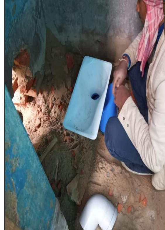
Retrofitting in progress
