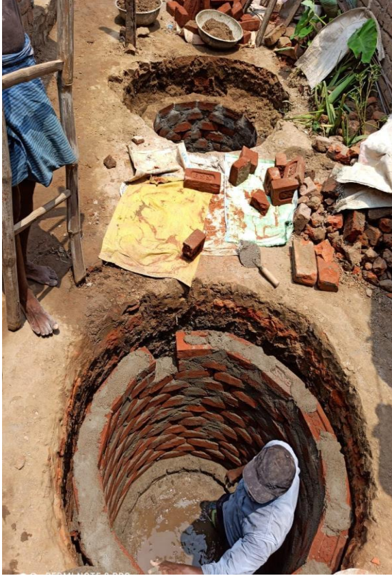
Retrofitting in progress
