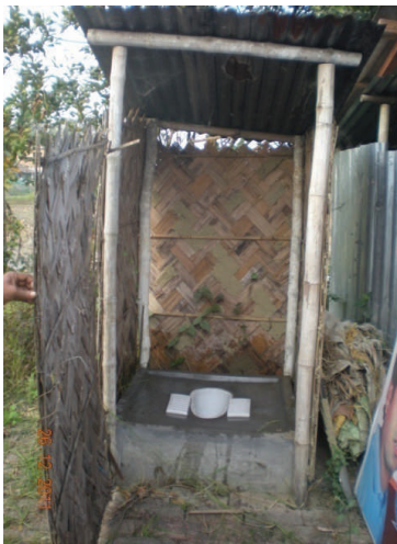
Supersaturate with thatch, and roof of G.I. sheet
