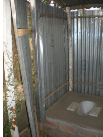
Superstructure with G.I. sheet
