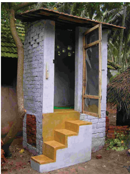
Ecosan toilet superstructure with brick, cement, and red stone roof and Tin door
