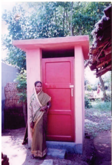
Superstructure with brick, cement and RCC roof and wooden door
