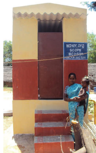
Ecosan toilet superstructure with brick, cement, and RCC roof and iron door
