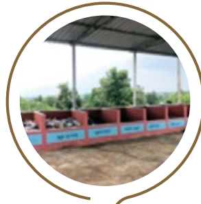
Secondary segregation at village level shed
