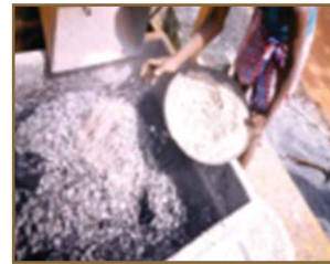
Shredded plastic being used in road making
