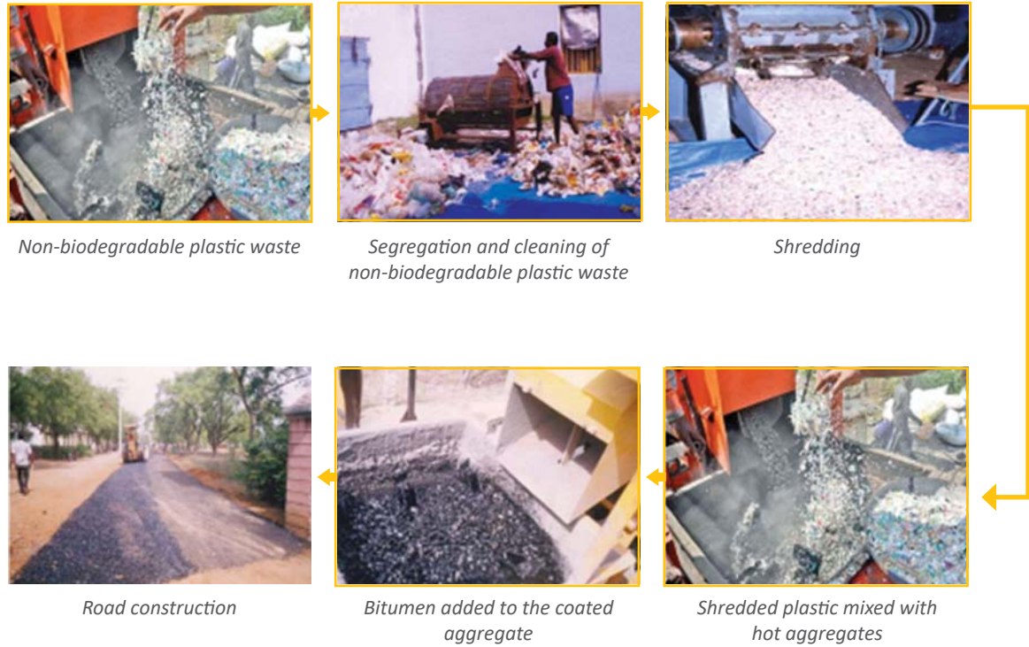
Figure 12: Plastic waste being used in road construction
