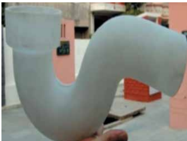
Figure 2A: An S trap or water seal
