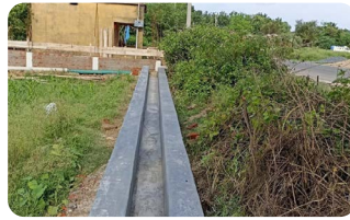
13,05,663 drainage facility sheds
