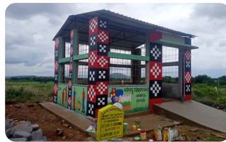
3,50,479 waste collection and segregation sheds
