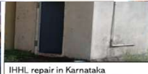
IHL repair in Karnataka
