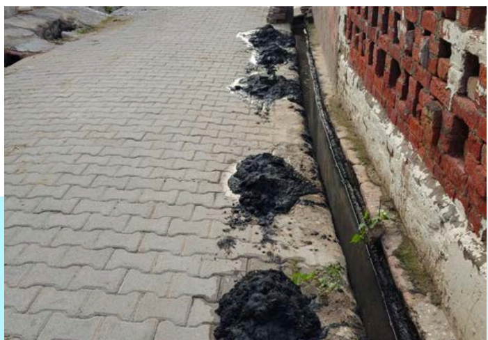
Drain Cleaning Drive under SHS 2026 – Haryana, Sonipat District, Sonipat Block, Kilorad Gram Panchayat.
