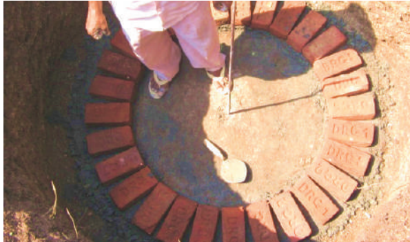
The first layer in 9" Brickwork
