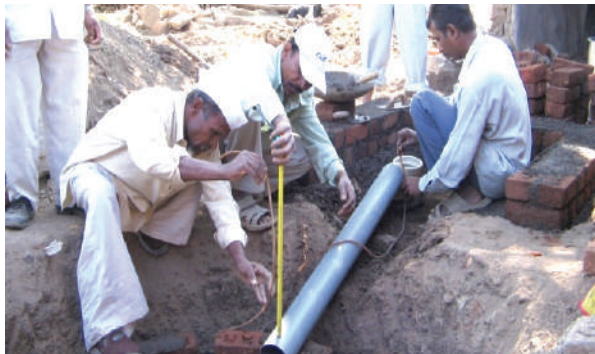
The pipe should have adequate slope
